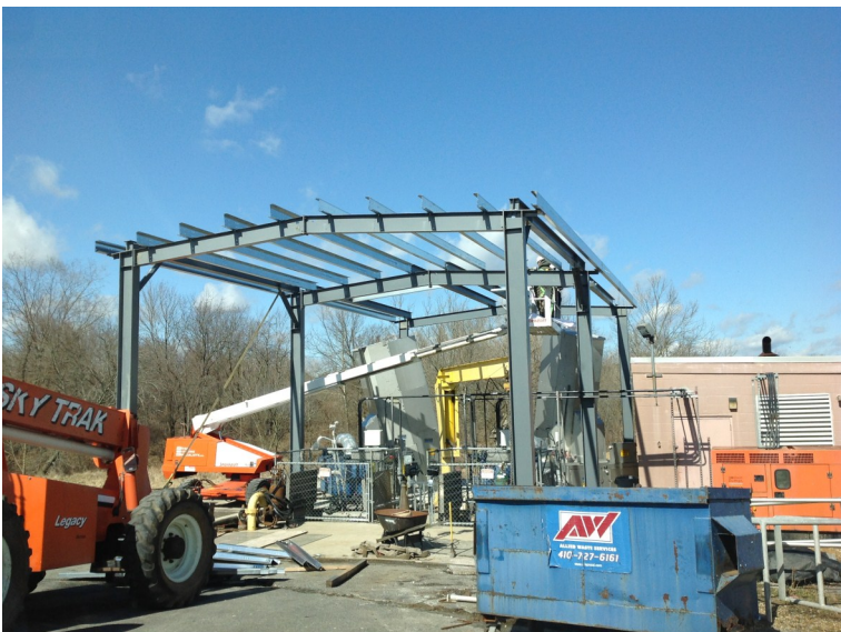
Structural Engineering –Dorsey Run WWTP - 2011
