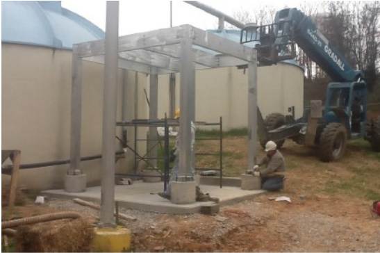
Structural Framing Inspection
