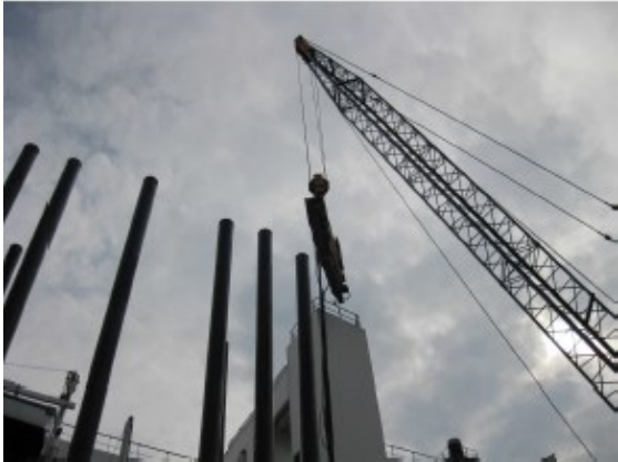
Inspection of Deep Foundation Installation
