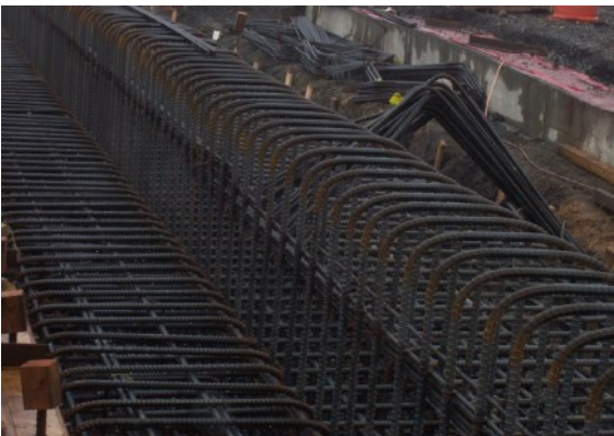
Concrete and Rebar Inspection
