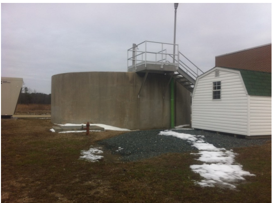
Eastern Correctional Institute Wastewater Treatment Plant Upgrade
