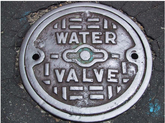
Engineering and GIS Support Services for Water Infrastructure Revitalization Programs
